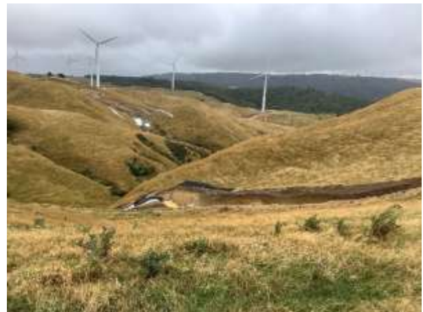
Figure 3. Sediment retention ponds in Construction Zone 2
