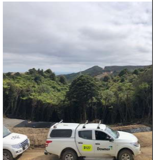
Figure 10. looking along southern access track/road
