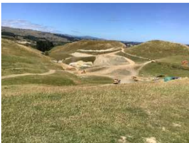
Figure 4. overview of construction Zone 1
