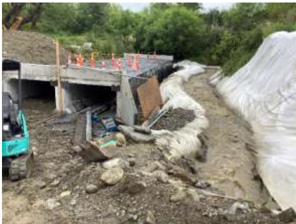
Figure 2. Temporary diversion as culverts are constructed off-line
