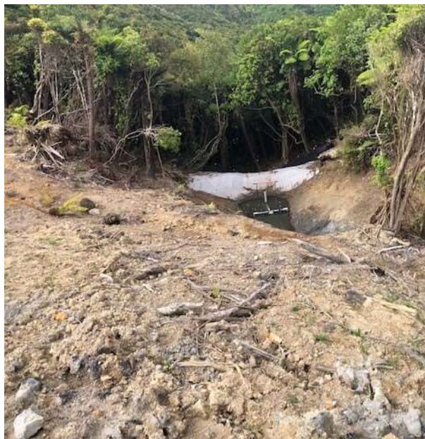
Figure 9. Decanting Earthbund installed in steep terrain
